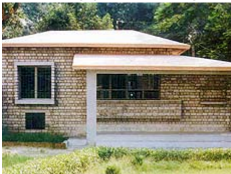
Flyash bricks produced locally.
