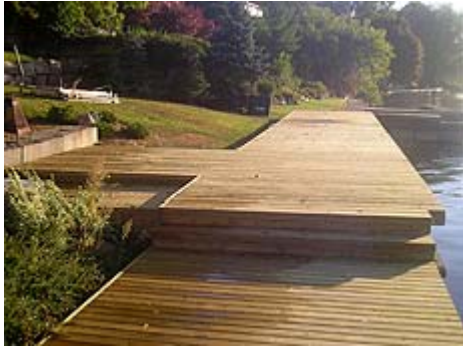
Recycled plastic used for building a pontoon.
