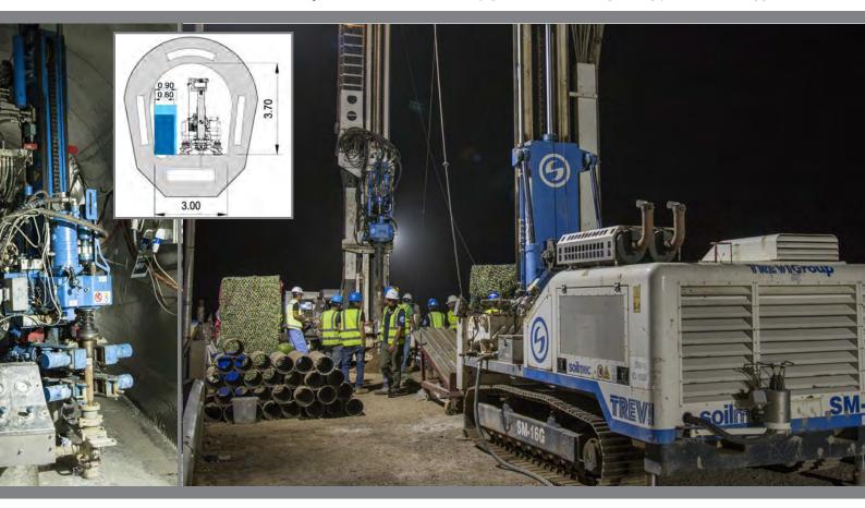
stability. For all cases, each borehole was pressure-grouted using a single packer, lowered in the hole at top of the stage to be grouted.
