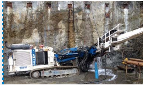
Temporary Ground Anchors: 30,000 m, Ø 165 mm anchors to the maximum depth of 30 m.
