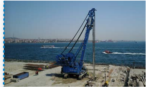
Diaphragm wall with HYDROMILL: 50,000 m 2 , 1200 mm thick panel to the maximum depth of 39 m.
