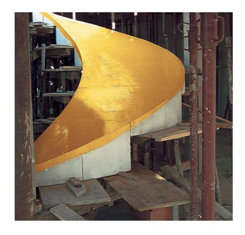
Formworks are produced in parts in order to facilitate handling in the building yard. Each element constitutes the bottom of two or more steps, depending on the size of the stairs. The forms are placed on a panelled falsework as required. The side supports are made up of vertical boards placed against the polystyrene on the sides of the ramp. Lastly, the boards for the rises are fixed to the sides like in traditional carpentry work.
