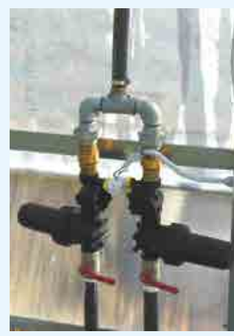
Double water-feeding group , ball valve, net filter and solenoid valve.
