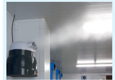
Humidifier in operation inside a germination chamber.
