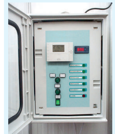
Remote control panel , for the timely management of temperature and humidity.
