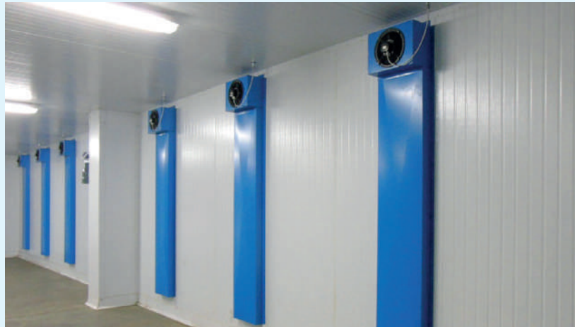
Electro-circulators for the temperature destratification inside chamber.
