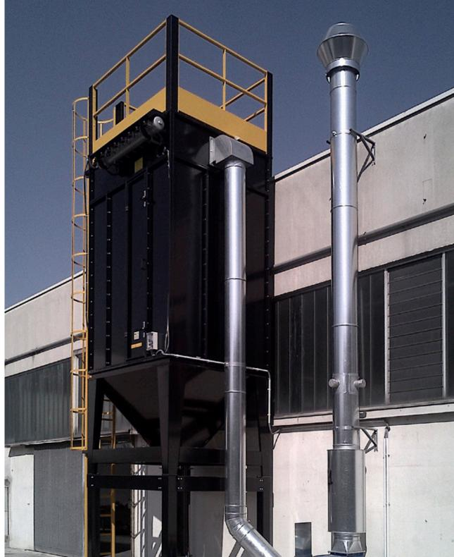
Horizontal sleeves filter-unit standard or with insulation
