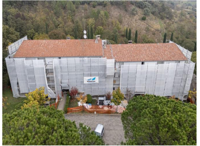
Condominium under envelope renovation — Renavitas site
