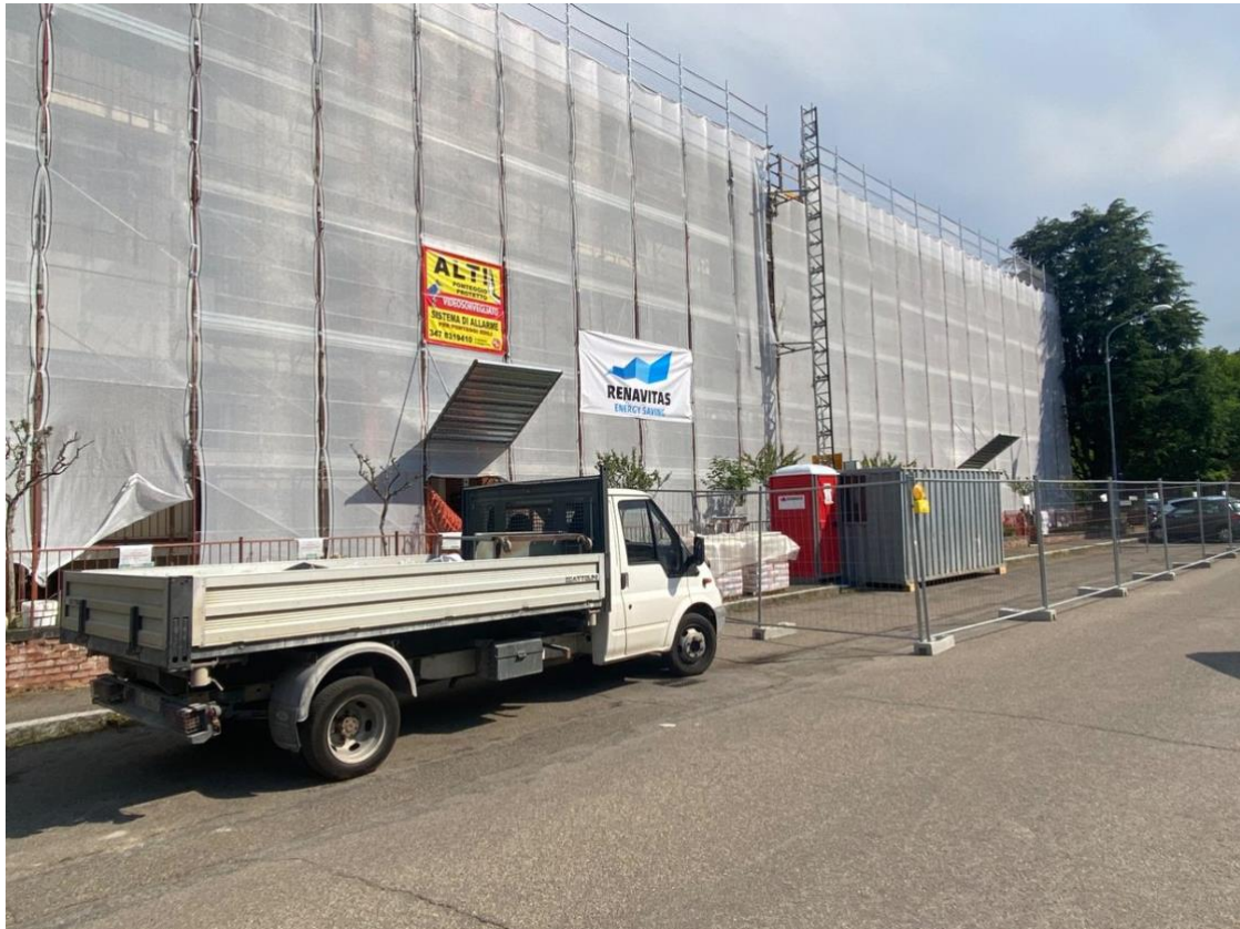
Active construction site — Renavitas full-envelope renovation, Emilia-Romagna
