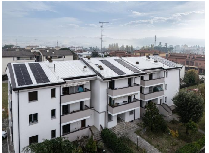
Multifamily condominium — PV retrofit on flat metal roof
