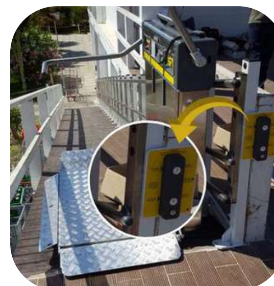
Fixed Control panel on the Landing
