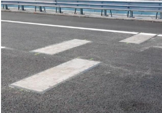
AISI 316L steel is in fact also suitable for extremely aggressive environments. The system also, in case of work on the road pavement is **easily repositionable** in a different site.
