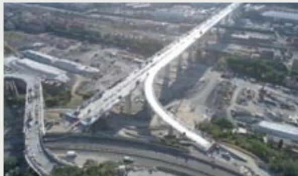
Genoa Saint George Bridge - Italy
