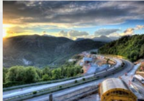
A3 Salerno – Reggio Calabria Highway - Italy
