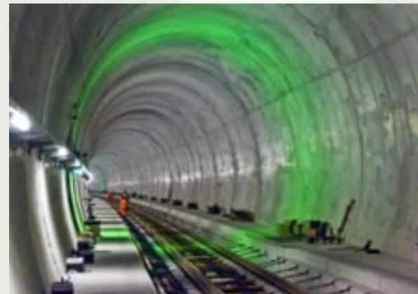
Monte Ceneri Base Tunnel - Switzerland
