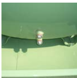
1" drainage point for routine maintenance and cleaning
