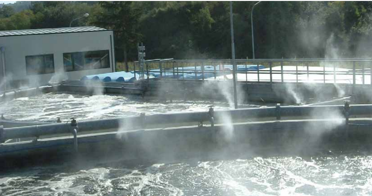
Outdoor diffused emission - 250 nozzles for wastewaters treatment
