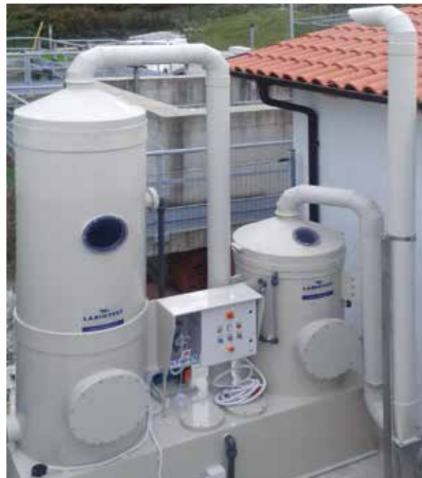
DkFil® + Scrubber applied to a wastewaters treatment plant.
