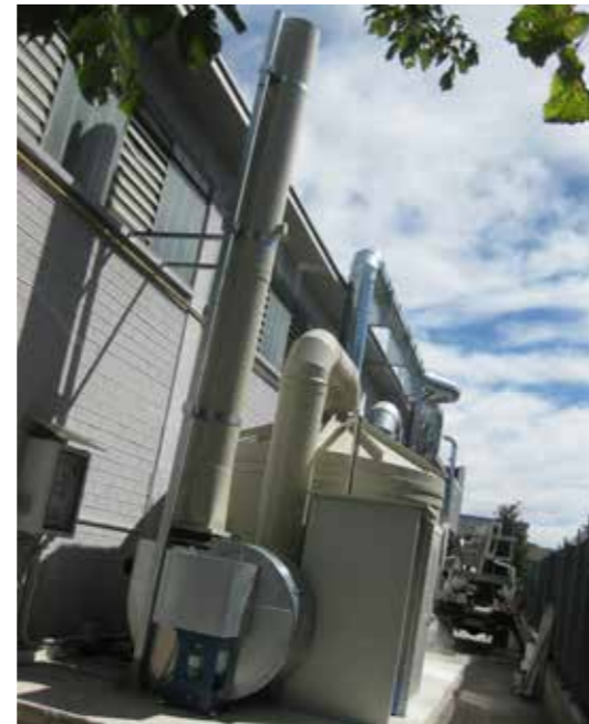
Application of an ultrasounds osmogenic barrier as an additional abatement step.
