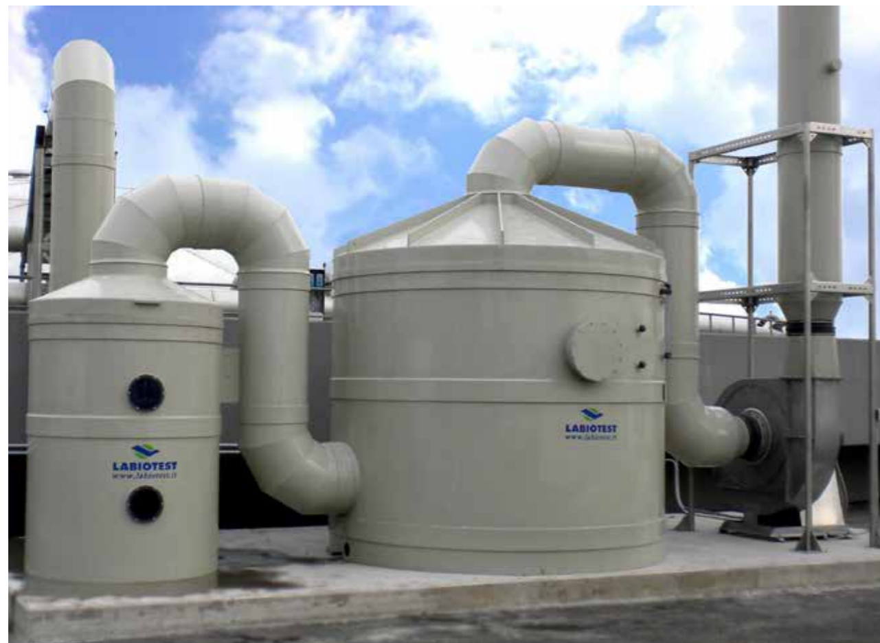
DKFil® 14.000 Nm 3 /h applied to a wastewaters treatment plant
