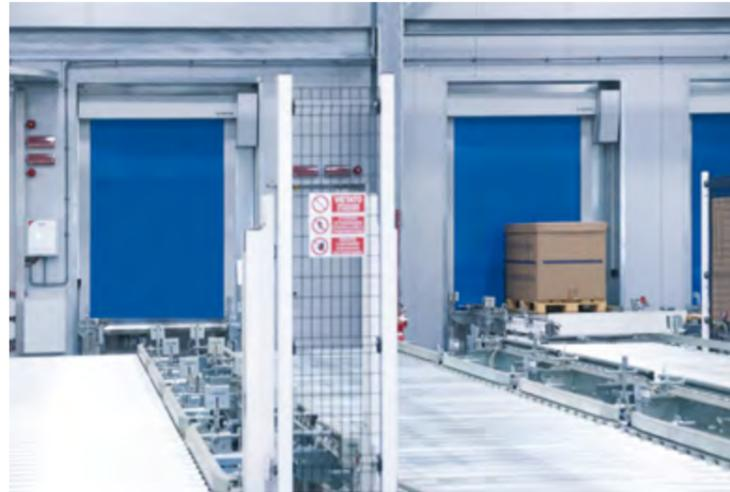
*ORS ( Oxygen Reduction System) doors find ideal locations in various industrial sectors and with different types of production, from food to cosmetics and pharmaceuticals , with the need to store goods safely . The doors fit perfectly into the automatic warehouse chain , separating the production areas from the storage areas. They are installed in environments with low oxygen levels. A very good fire extinguishing system.*
