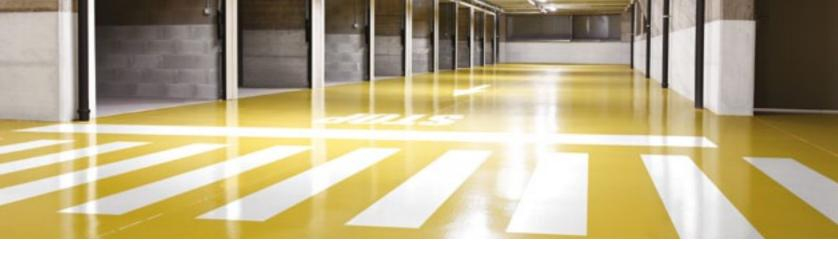
Parked cars deposit liquid residues such as water, oil and fuel on the floor. It is therefore advantageous, for this kind of flooring, to rely on waterproof and chemical-proof materials, which allow to have durable horizontal signposting, skirting and chromatic differences between different parking areas.
