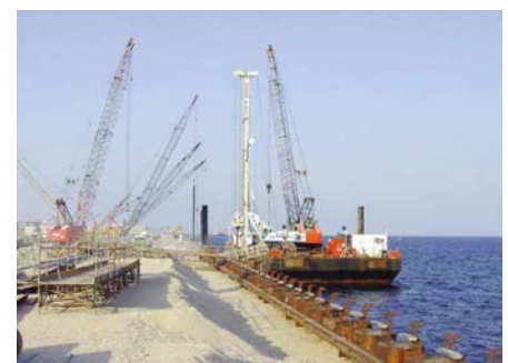
Q. Chem Petrochemical Complex_Qatar
