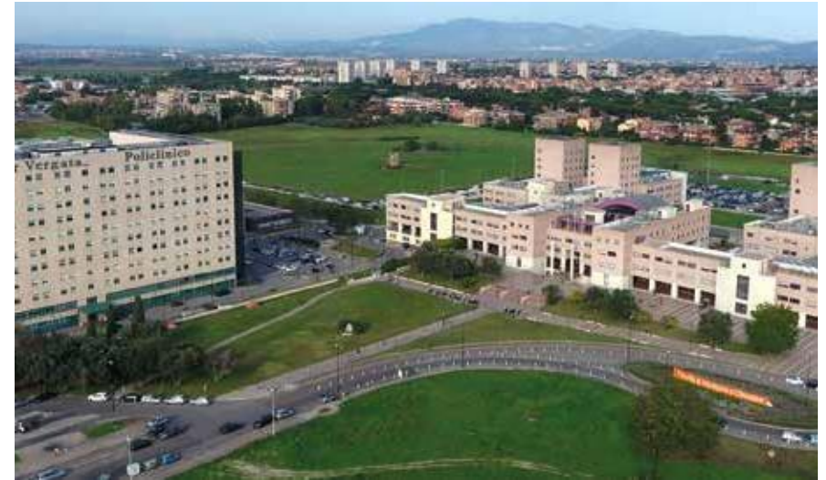
Tor Vergata University in Rome: thermal power plant
