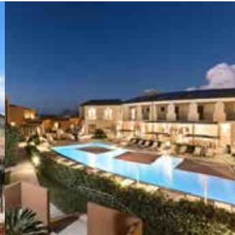
TERRADIMARE RESORT&SPA SAN TEODORO, ITALY
