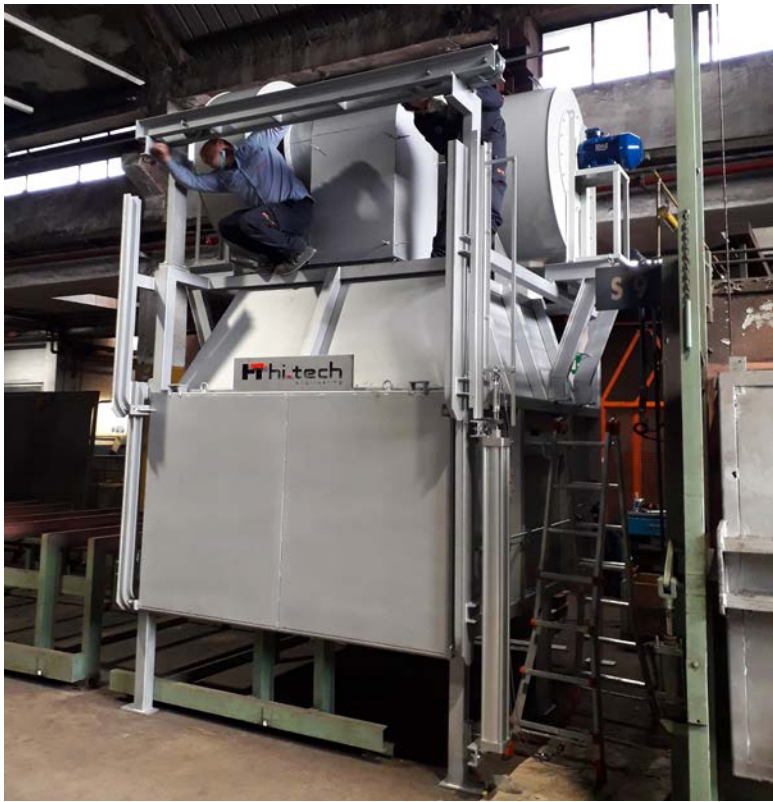
Revamping of modular line with new isothermal cell.
