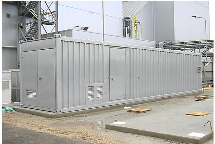
TM containers can be moved with cranes through upper and lower corner casting.
