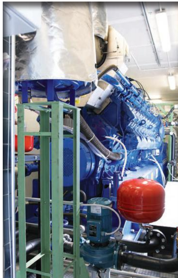
> Inside view of a REC 2000 unit
