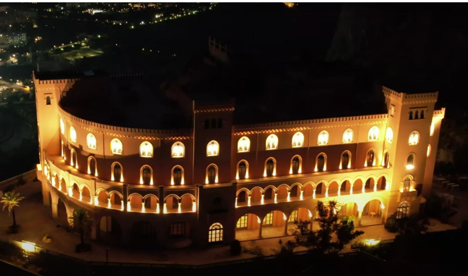
Utveggio Castle - Energy efficiency intervention with application of the RasoThermo + Reflex-out cycle.
