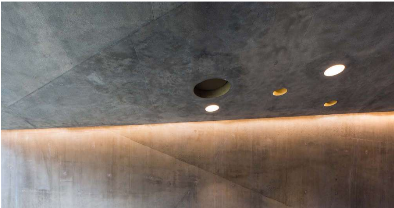
New church and pastoral center Cavernago (BG) Detail of the concrete ceiling
