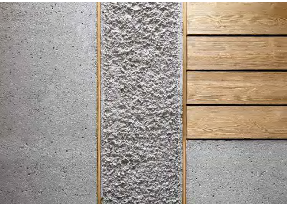
New Church in Carpi (MO) Detail of the different surfaces used in the church interiors.
