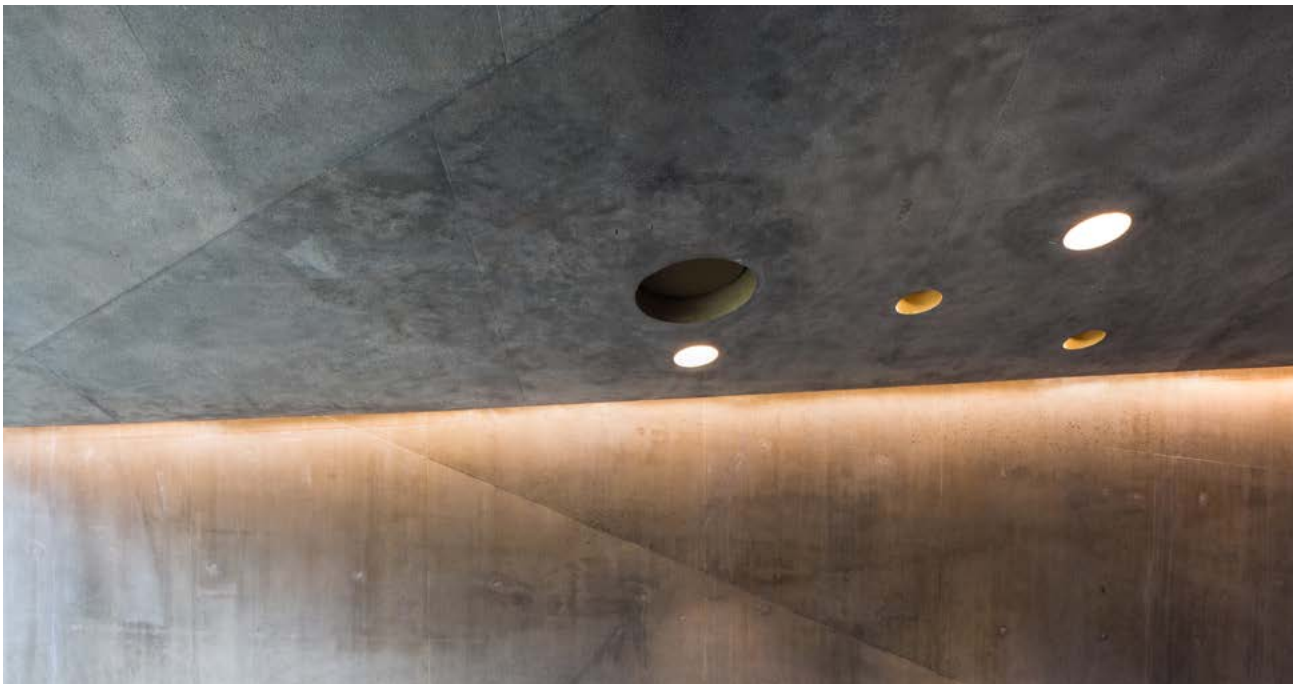
New church and pastoral center Cavernago (BG) Detail of the cocncrete ceiling
