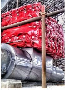
SIPA is a leading manufacturer of passive fire protection systems. Our flexible covers called MATTFLEX SIPA ® are designed to insulate equipment and delay temperature rise in the event of a UL1709 and ISO 228997 hydrocarbon jet fire scenario. MATTFLEX SIPA ® has Type approval certificate and includes innovative simulation software.
