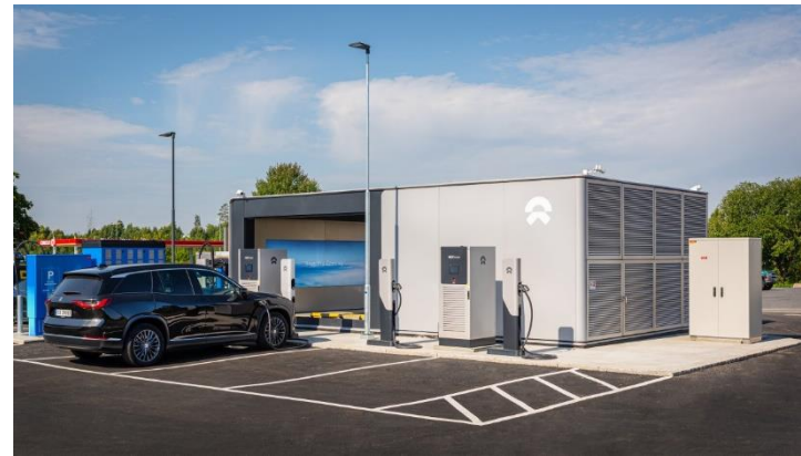
Norwegian swappable battery station (Source: NIO)
