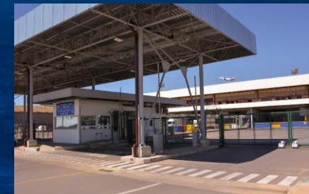
Access gate with security control
